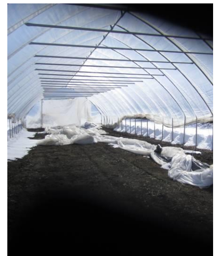
Fig. 2. Gothic tunnel following a heavy snow event in early spring of 2015.
