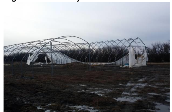
Fig. 2. Wind damage to cover of Gothic high tunnel over winter of 2013/2014.
