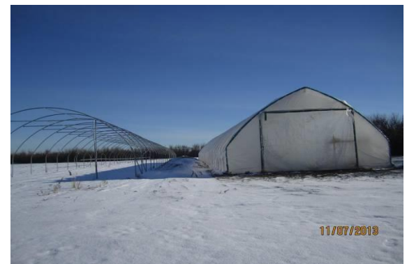
Fig. 2. Gothic (right) and supersolo (left) high tunnels in early winter of 2013/2014.
