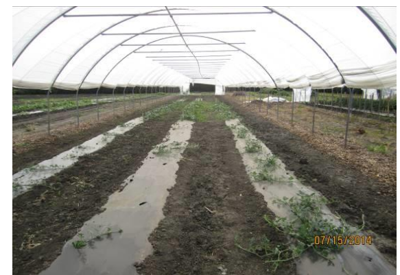
Fig. 2. Wind damage to cover of Gothic high tunnel over winter of 2013/2014.
